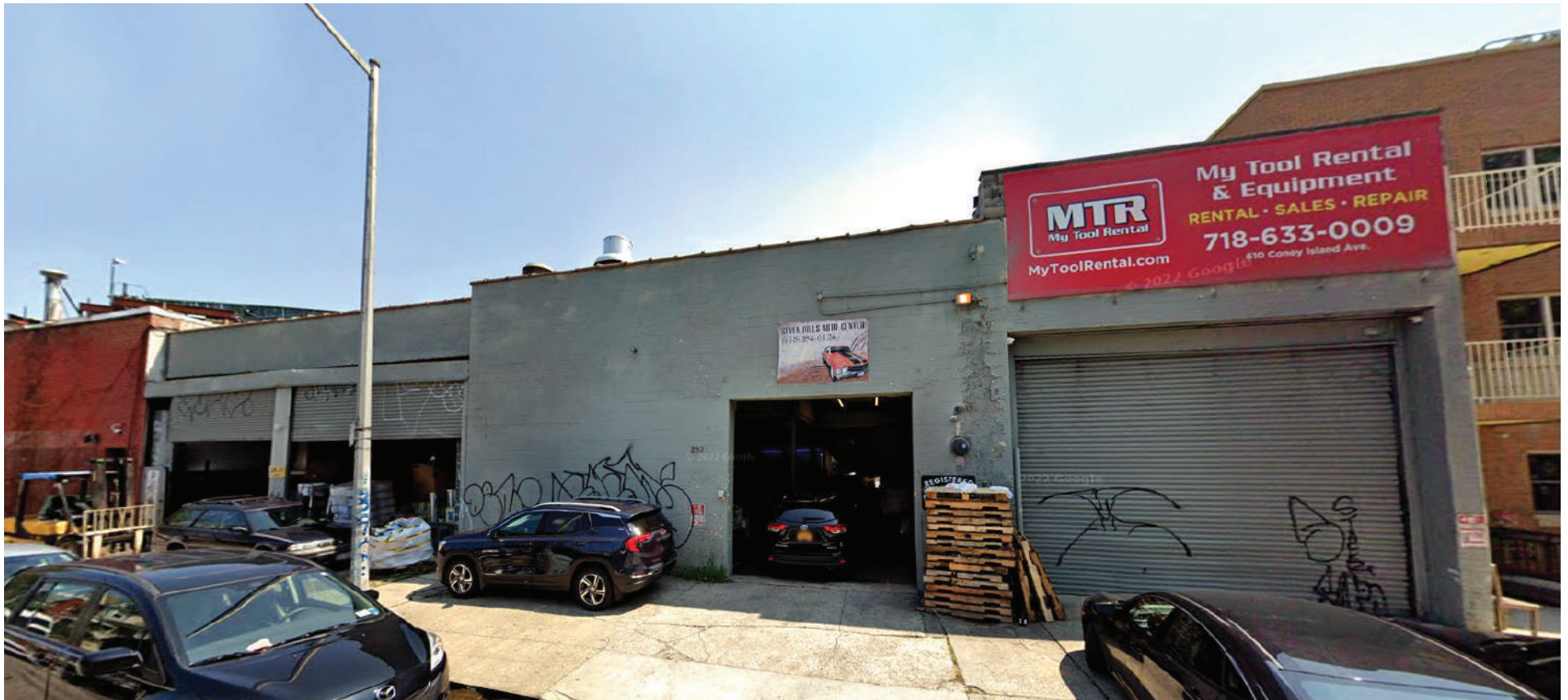
BACK OF BUILDING LOCATED ON EAST 9TH STREET
