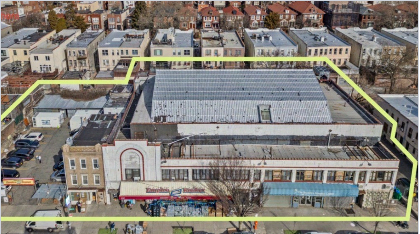
The existing building at 529–547 Empire Boulevard — ±32,900 SF across three stories, with grade-level frontage on Empire Boulevard, private parking and rear access via the Montgomery Street laneway.
